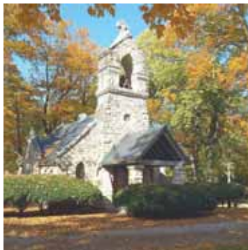
St. John the Baptist Chapel (ca. 1890), on the Old Gillett Farm.
