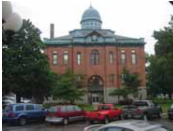
Menard County Courthouse (1896).
